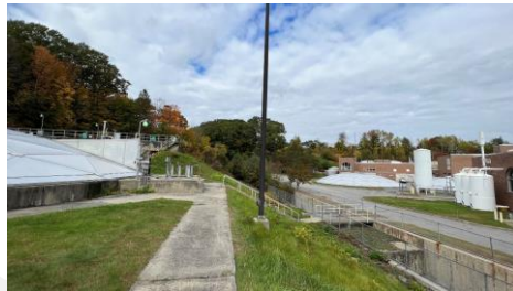
Figure 1 - Augusta WWTF Site - note secondary facilities on left at higher elevation
