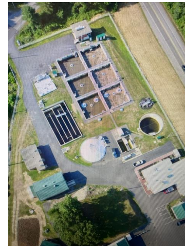
Aerial View of Kittery's Wastewater Treatment Facility
