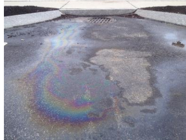
Figure 3: petroleum products entering the stormwater system
